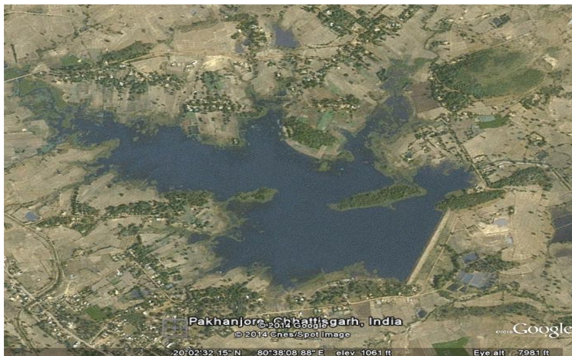
Figure-1. Satellite image of Pkhanjore Dam
